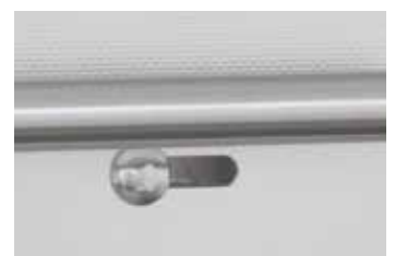
Adjustable air inlet integrated in the door
