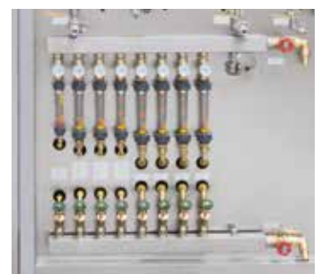
Cooling water distribution
